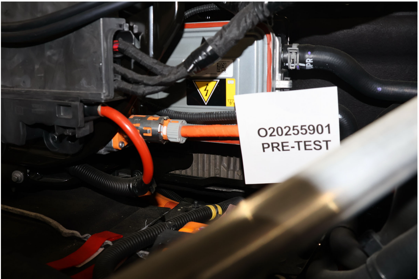
Photo No. 305-02 - Power Inverter Warning Label
